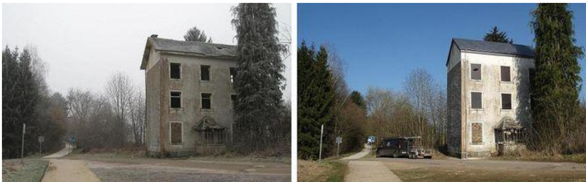
Figure 22. Before and after photographs of the old guard house in Virton
