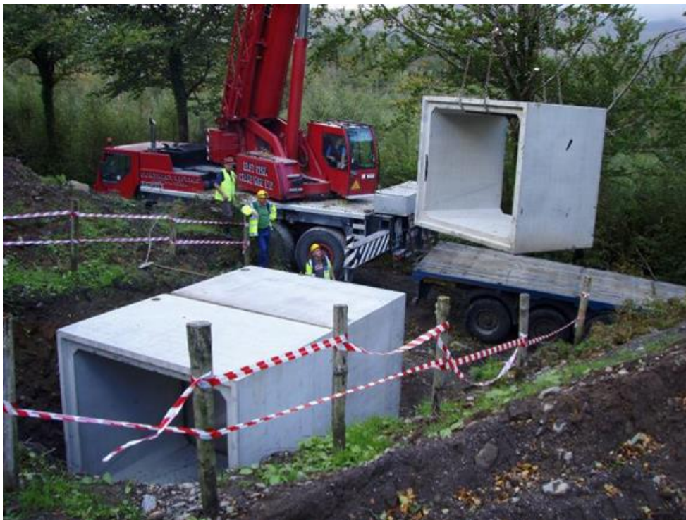
Figure 30. Square profile pre-cast concrete sections being loaded into place.
