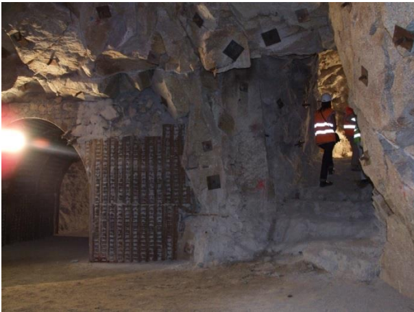
Figure 21. Galleries for the bats to roost in
