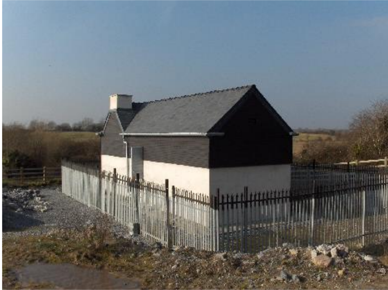
Figure 2. The Ennis bat house shortly after construction.
