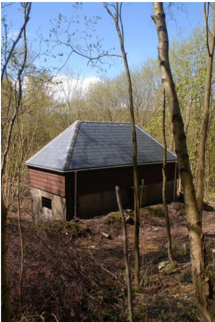
Figure 25. The completed conversion to a bat house
