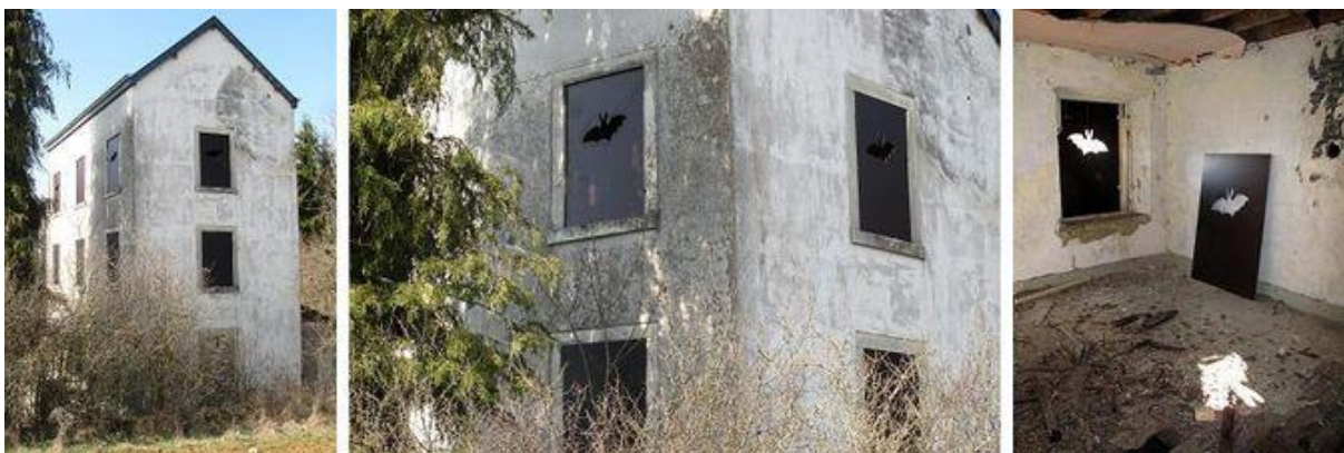
Figure 23. Photographs of the shutters and bat access holes
