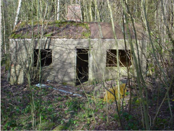
Figure 24. The derelict mine wages office
