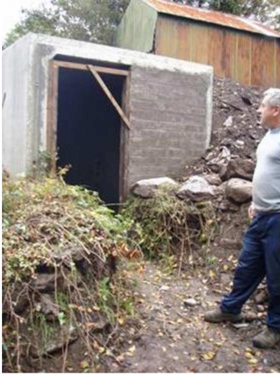
Figure 31. The new hibernation site before it was covered in earth
