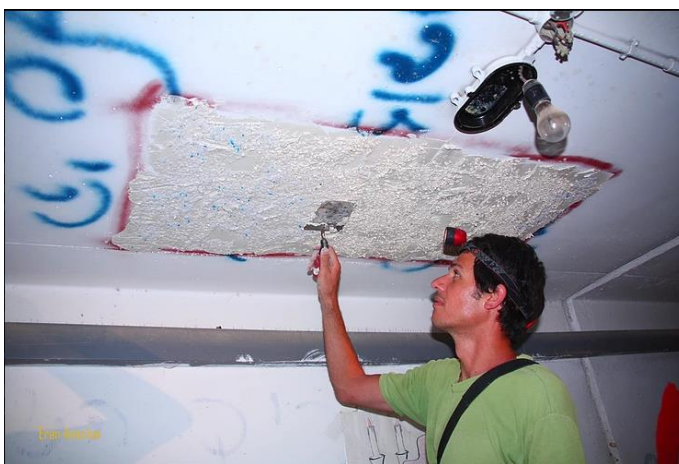
Figure 28. Roughing up the smooth ceilings
