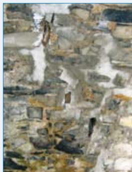
Figure 22. Underside of Lisconny Bridge; showing the three sections of the deep fissure that were left open to accommodate the nursery colony of *Myotis daubentonii*. The nursery roost is located in the lowest section. Note how the stonework was carefully grouted around and not over.
