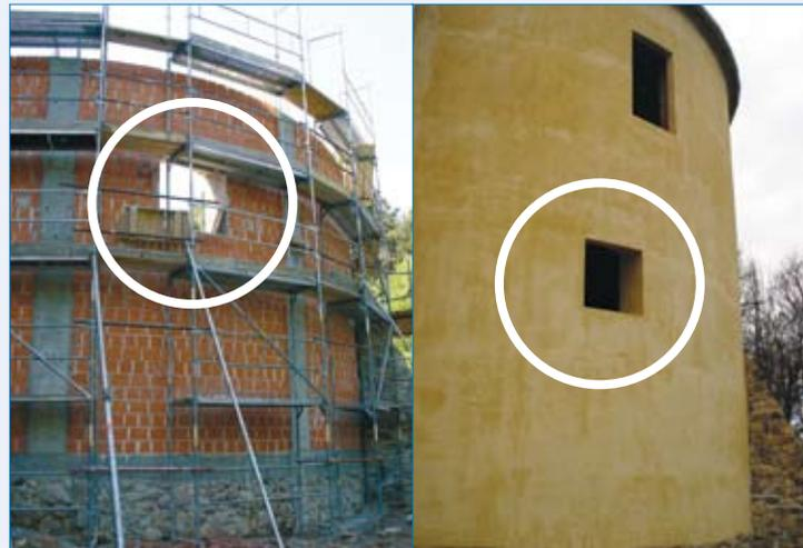
Figure 16. Northwest tower of Grad na Goričkem castle, Slovenia, during and at the end of reconstruction in year 2006 (circles mark new entrance openings for bats).
