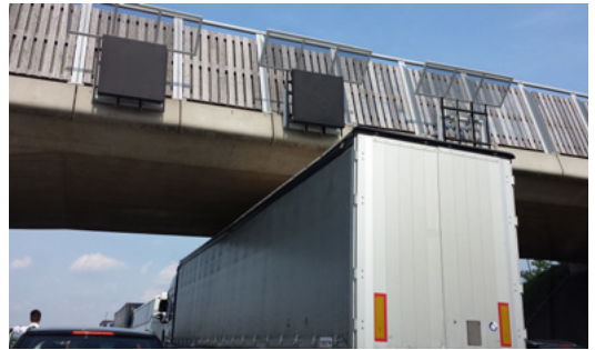
Figure 5.6. In the Netherlands, walls were designed to avoid light trespass from a highway to a wildlife bridge with commuting routes (© H. LIMPENS).
