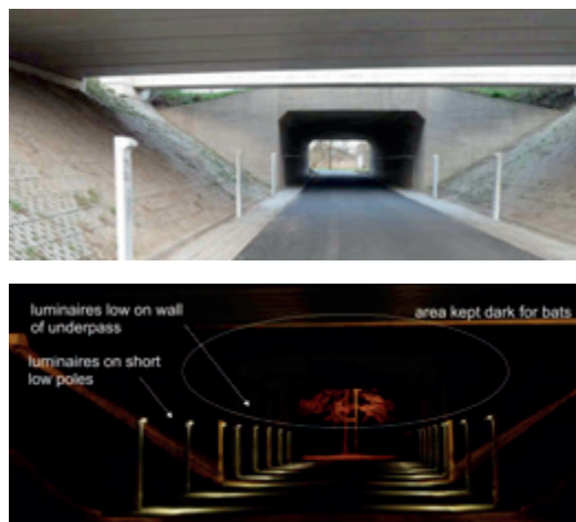
Figure 5.3. Installation of luminaires on short poles for mitigating the effect of ALAN on a commuting route through an underpass in the Netherlands (the same place in daylight and at night). This solution was proven as efficient for P. pipistrellus but not for the low-flying species M. daubentonii (© F. BREKELMANS).
