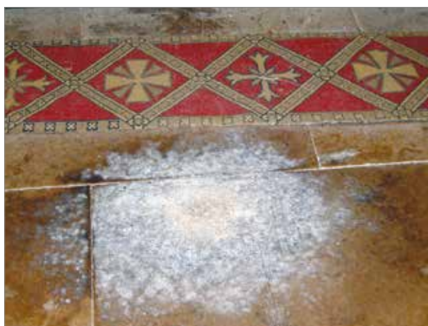
Figure 13. Damage to stonework at Penmon Priory, Wales, United Kingdom, due to long-term exposure to bat urine.
