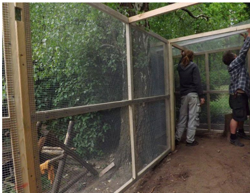
Fig. 3.*. Constructing the bat aviary.
