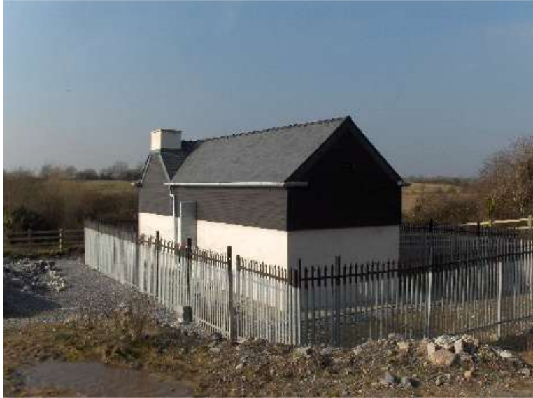
Figure 2. The Ennis bat house shortly after construction.
