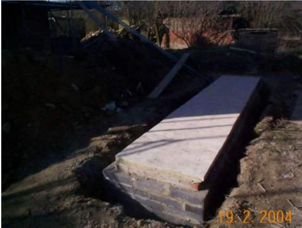
Figure 33. Part of the blockwork tunnel system connected to the maternity roost before it was covered over with earth
