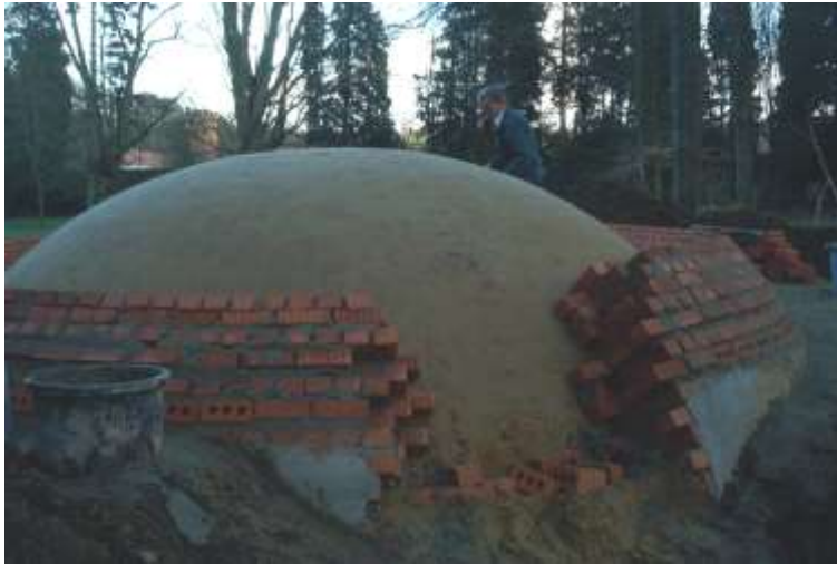
Figure 38. The brick dome being built over the straw and sand forma.
