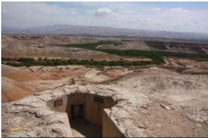
Figure 27. Entrance into the modified bunkers
