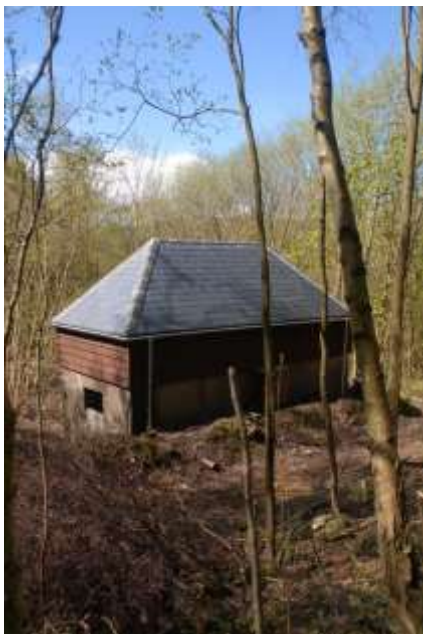
Figure 25. The completed conversion to a bat house
