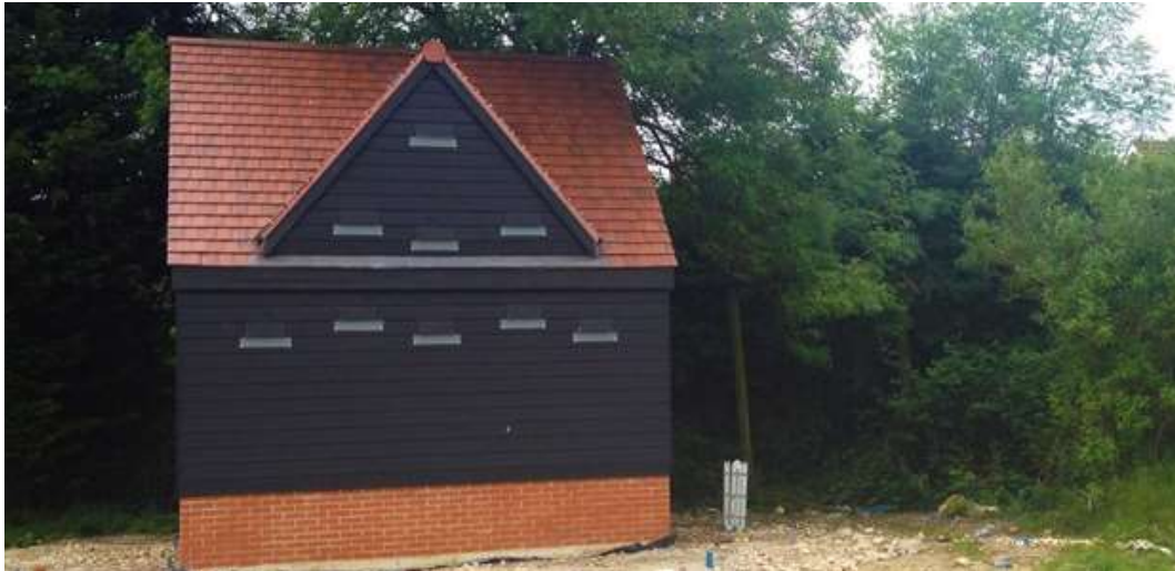
Figure 11. New built roost for Plecotus auritus with slot entrances for crevice dwelling bats.
