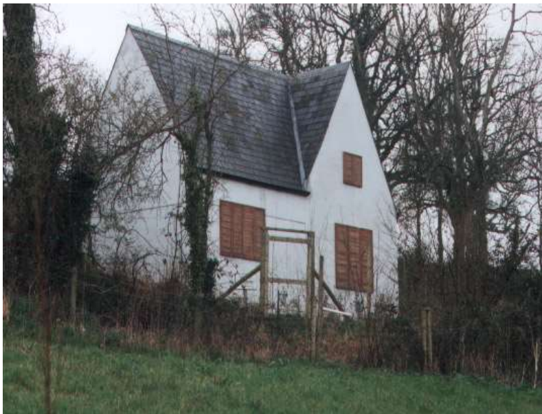
Figure 1. Bellaire Bat House. The false shutters were added to this building after construction to make it look less conspicuous.
