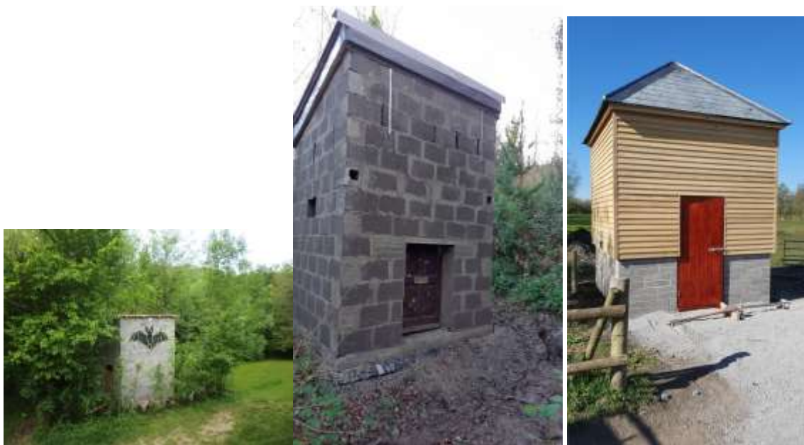
Figure 10 Bat towers constructed for Rhinolophus hipposideros in France (left) Ireland (centre) and UK (right)
