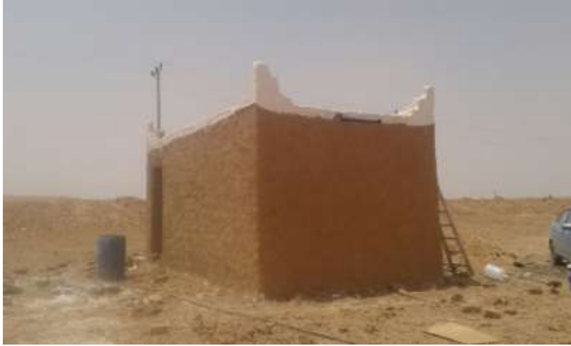
Figure 18. Newly constructed mud brick bat house.
