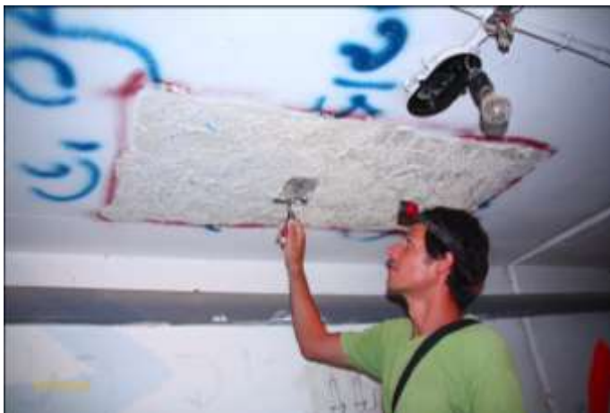
Figure 28. Roughing up the smooth ceilings
