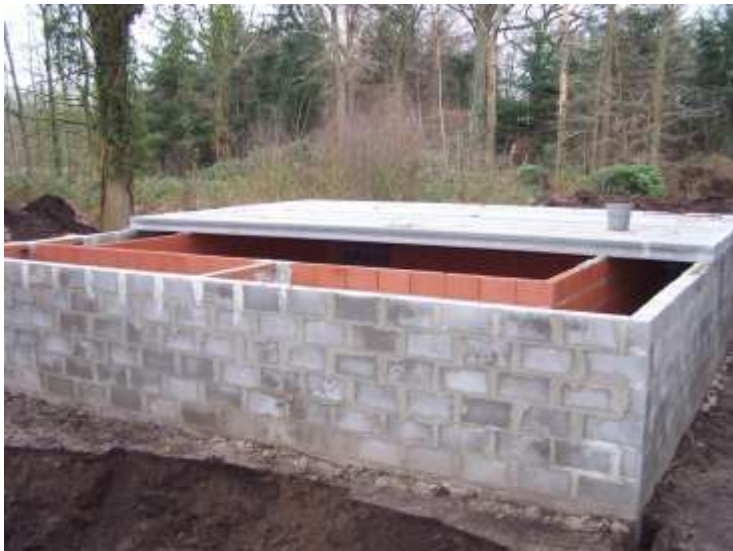
Figure 35. Showing the solid concrete walls and the lighter internal one.
