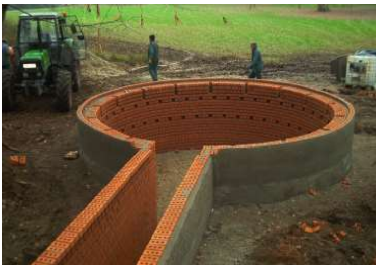
Figure 37. The Bulskampbeld hibernation site part way through construction
