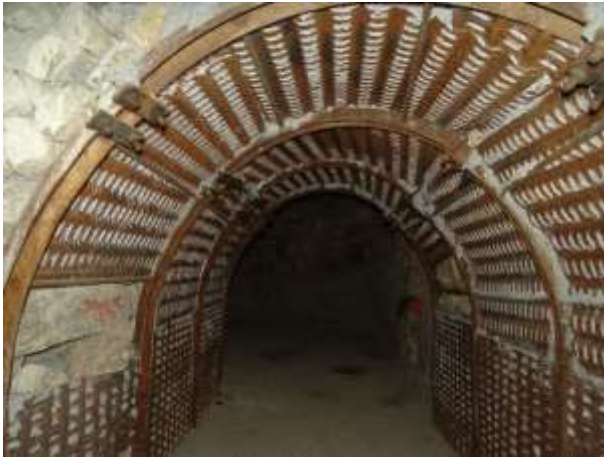
Figure 20. Excavated tunnel in the replacement roost
