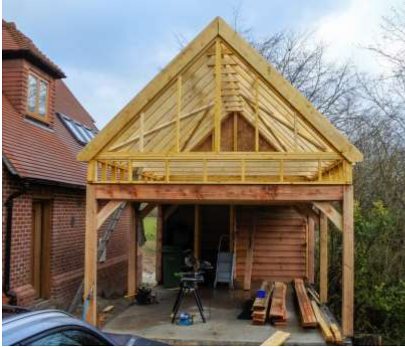
Figure 13. A dual use building with a garage below and bat roost above.
