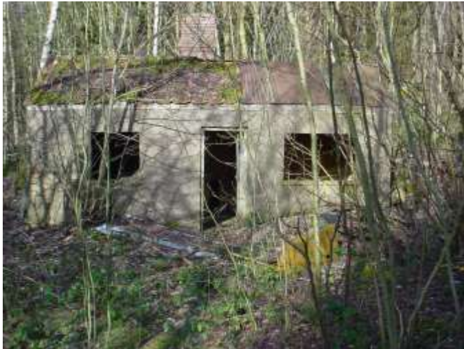
Figure 24. The derelict mine wages office
