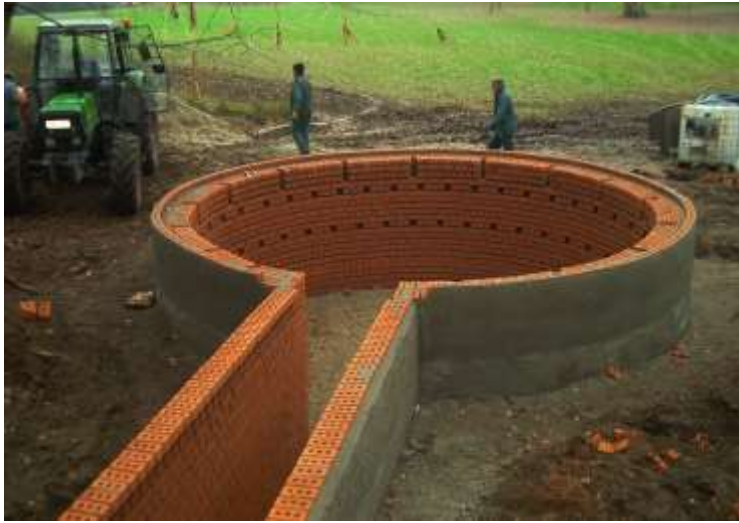
Figure 35. The Bulskampveld hibernation site part way through construction
