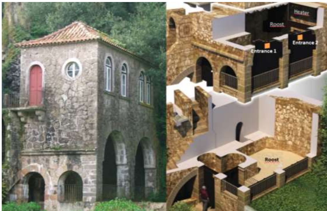
Figure 24. A photograph of the new roost building, along with a cutaway graphic showing the location of the roost, the entrances and the location of the heaters.
