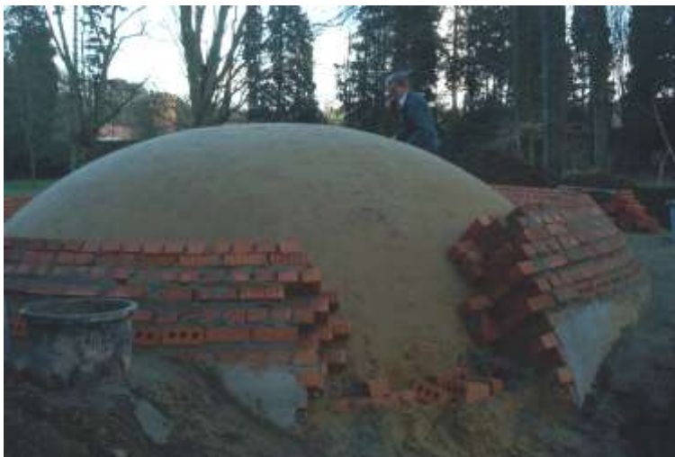
Figure 36. The brick dome being built over the straw and sand forma.
