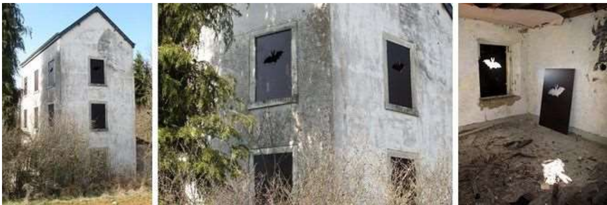
Figure 21. Photographs of the shutters and bat access holes
