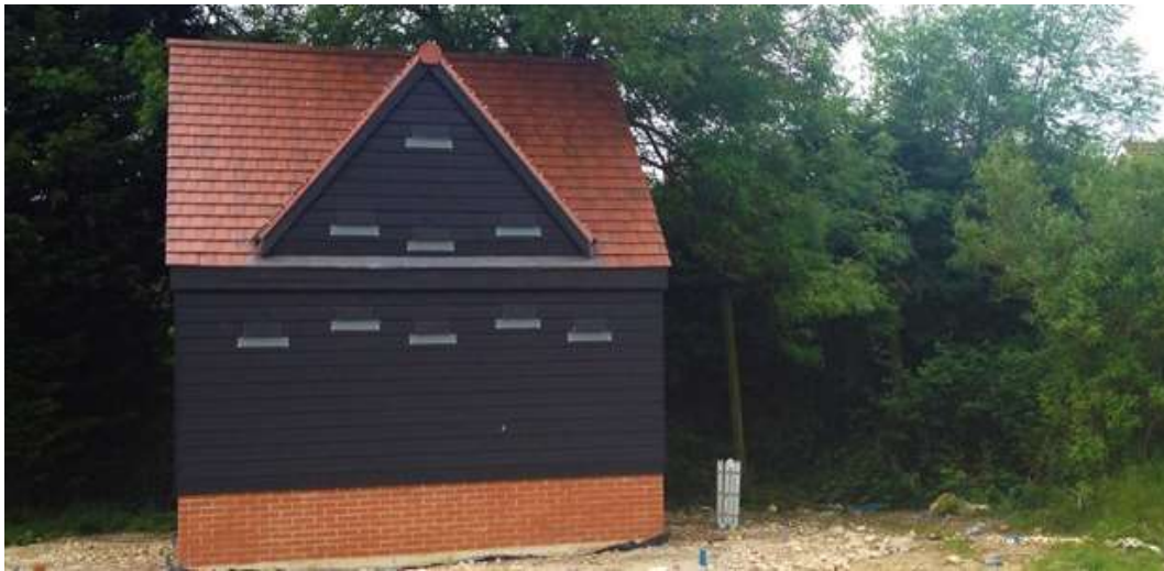
Figure 10. New built roost for Plecotus auritus with slot entrances for crevice dwelling bats.
