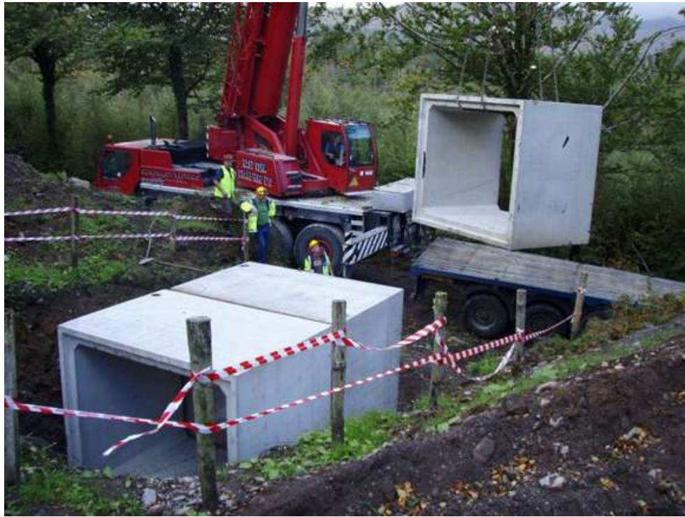
Figure 28. Square profile pre-cast concrete sections being loaded into place.
