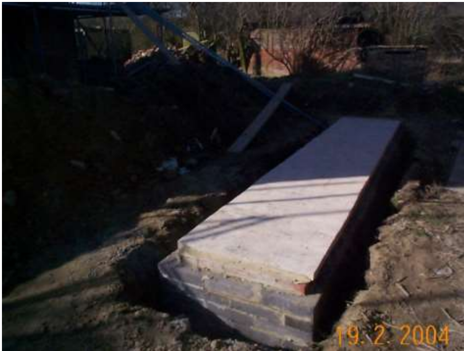
Figure 31. Part of the blockwork tunnel system connected to the maternity roost before it was covered over with earth
