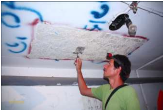
Figure 26. Roughing up the smooth ceilings
