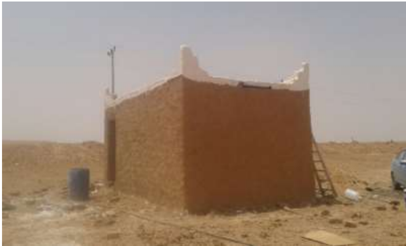
Figure 16. Newly constructed mud brick bat house.
