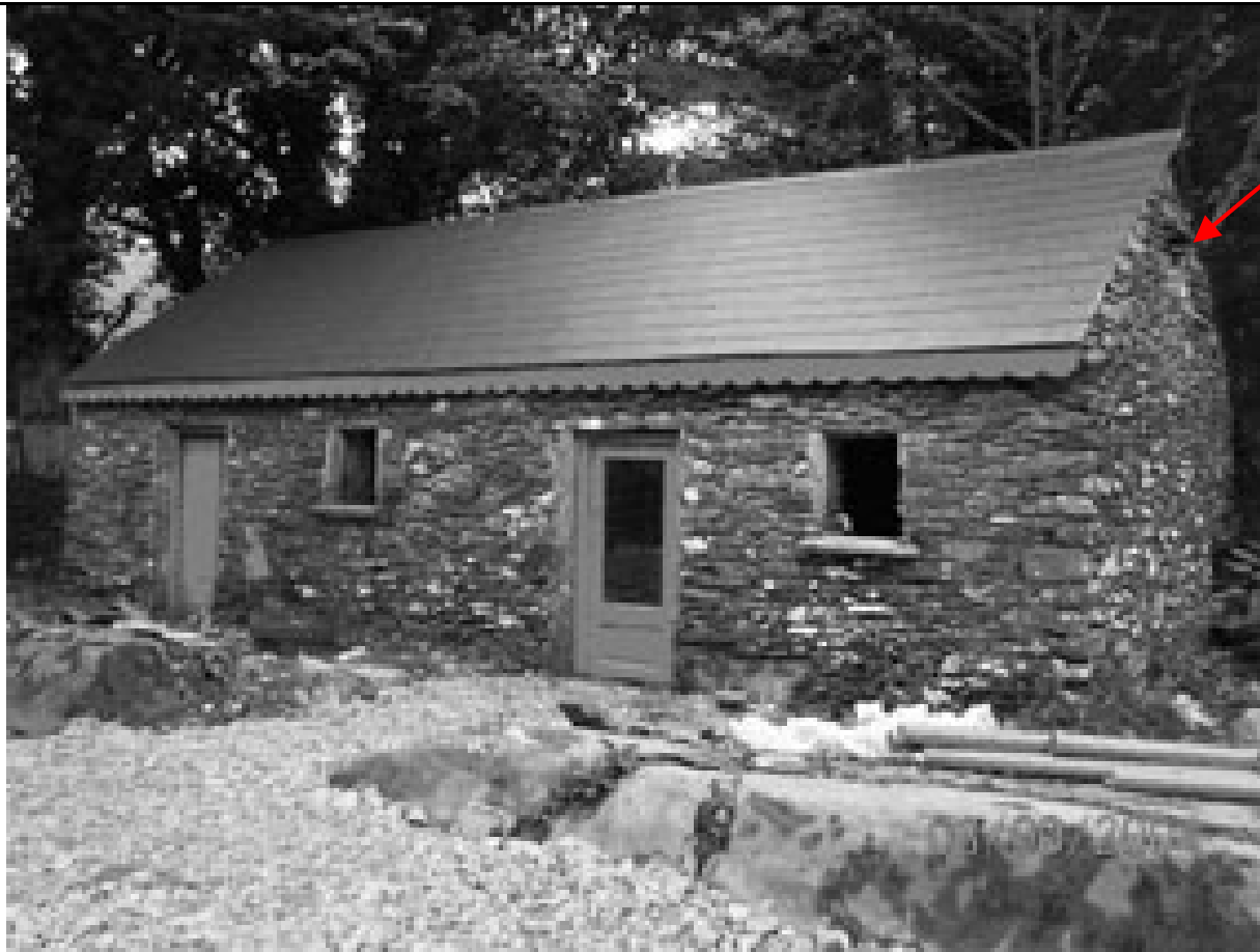
Outbuilding at Glaninchiquin renovated to allow lesser horseshoe bats roost in the attic. Arrow indicates access point made for bats into attic space.
