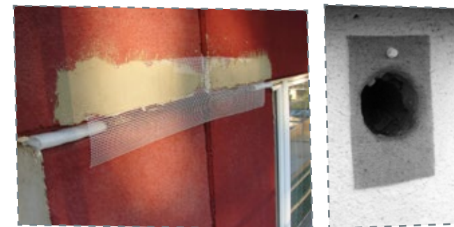
One-way closure using a curtain made of a light wire or plastic mesh, fixed only above the opening or fissure. It must not be loose and should overlap the opening sufficiently at all sides.
