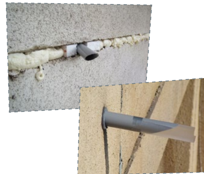
One-way closure using a sloping smooth metal or plastic pipe. The pipe should be slanted downward and protrude from the wall by at least 10 cm.
