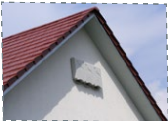
The summer & winter woodcrete bat box by the German company Schwegler, installed on facade surface, may be used as an interesting architectural feature.
